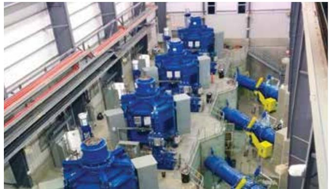
*Powerhouse - 4x6 jet vertical shaft pelton turbines*
